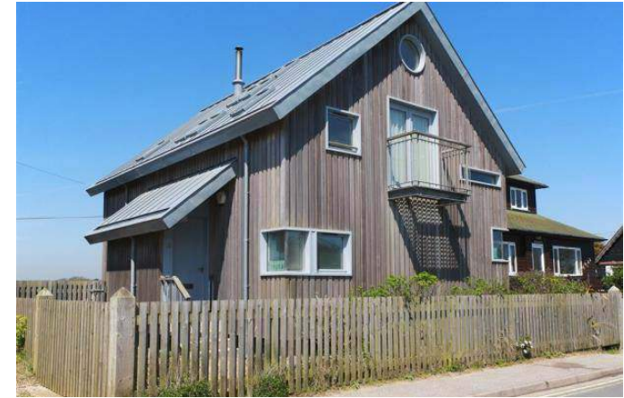
Ferryway, Ferry Road, Southwolk
